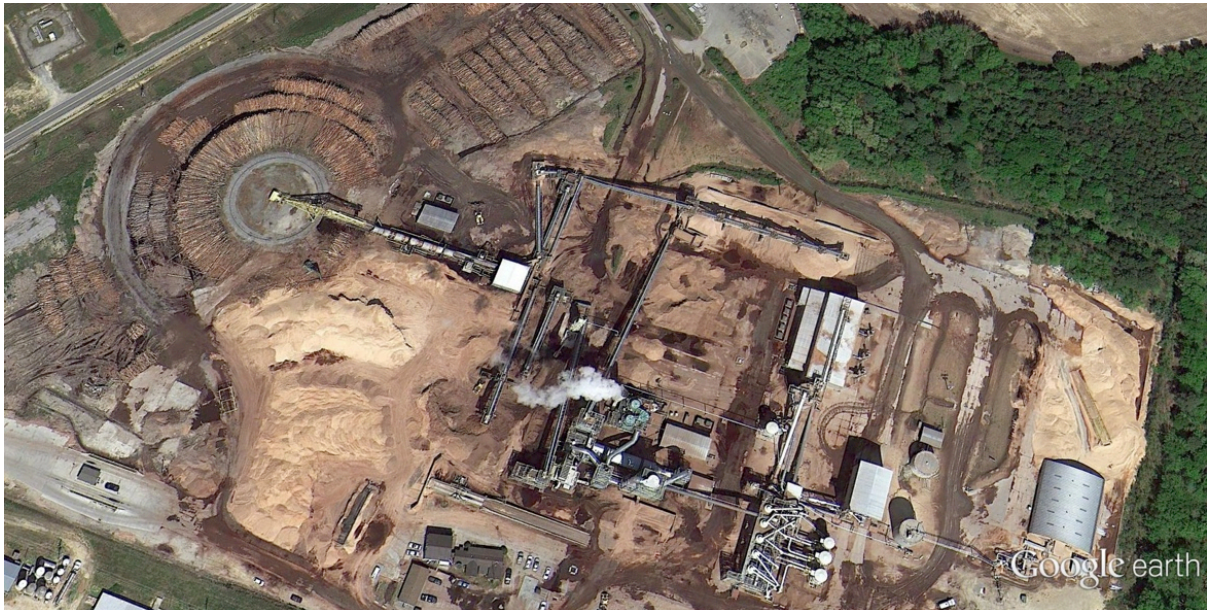
Photo: The Enviva pellet mill in Ahoskie, NC. On the left, raw materials can be seen: low quality logs as well as saw dust and chips. Being located in a region with both short rotation industrial plantations as well as native bottomland hardwoods. The sourcing of this and similar facilities has come under heavy scrutiny (Hammel & Smith 2013) and could be impacted by EU biomass sustainability criteria.
