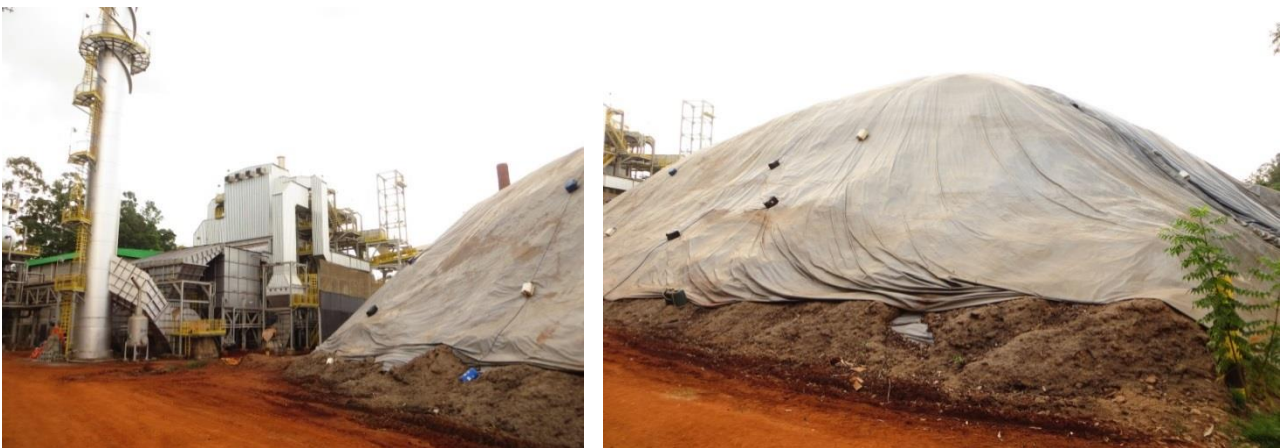
Figure 20 - Left: steam boiler for firing bagasse, Right: stored leftover bagasse from previous season. Araras, São Paulo
